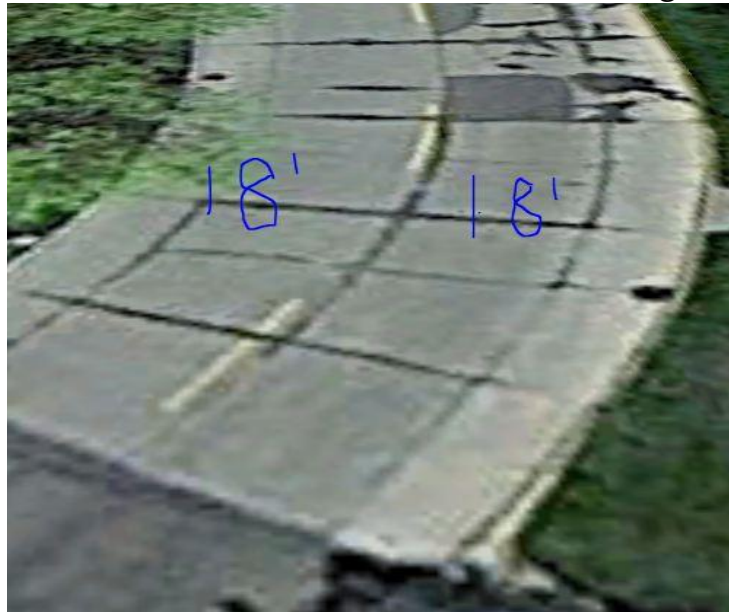
Figure 1: Pelham Boulevard lane widths from River heading Northward
