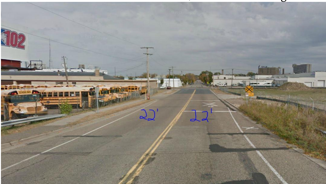
Figure 7: Pelham Boulevard lane widths, north of I-94 bridge
